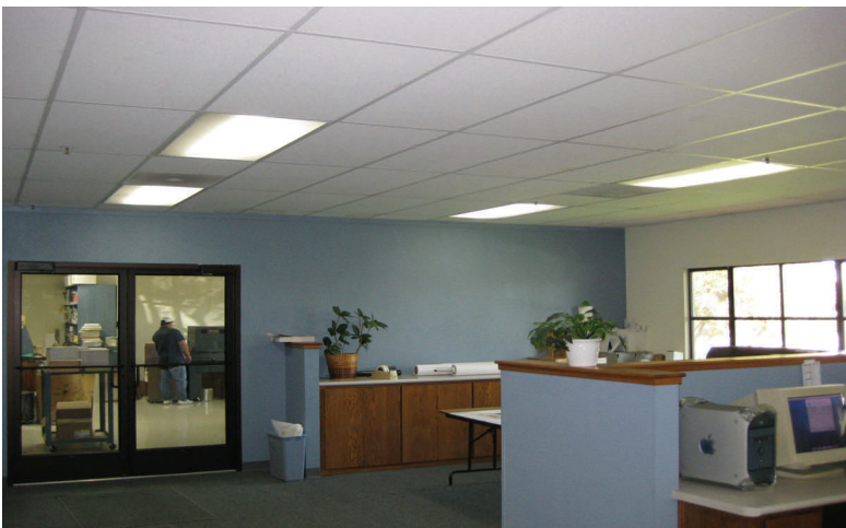
Wall mounted controls allow the employees to select the desired level of lighting. Here, only one lamp per fixture is on .
